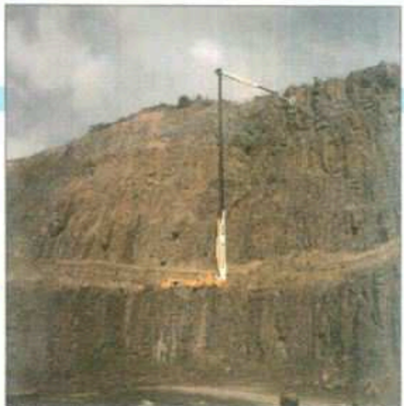
Safety survey of quarry face.
